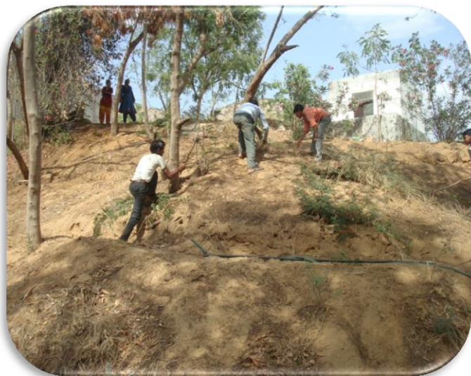
Stabilizing sand dunes through bench terraces and contour trenching
